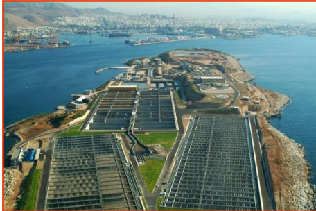
Athens Water Company SA (EYDAP SA) Psyttalia Waste Water Treatment Plant (Athens 2011 - 2014)
